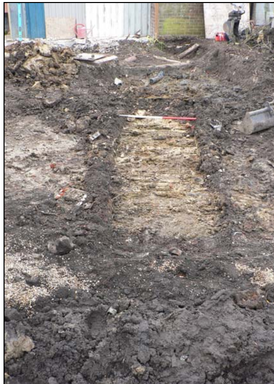
Trial trench across link extension area
