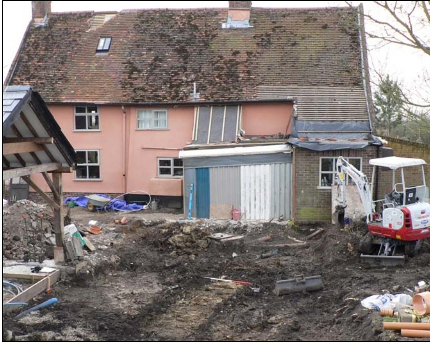
Link extension area from north
