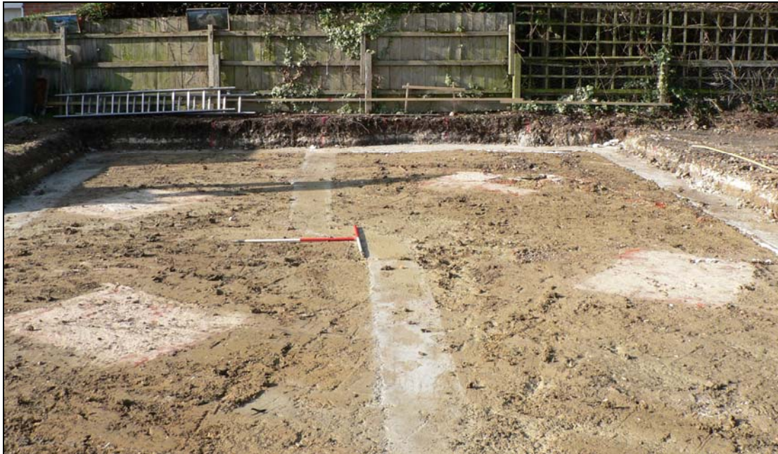
4. Brick pier bases from east
