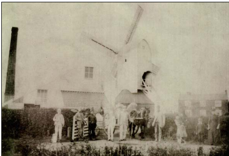
Frontispiece: Photograph of Naughton Mill from south c1900 (Mill House to right background, chimney for later steam to left, web source 1)
