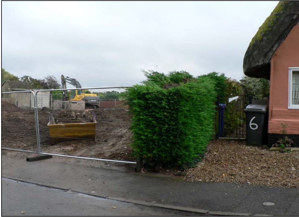
General view from southwest
