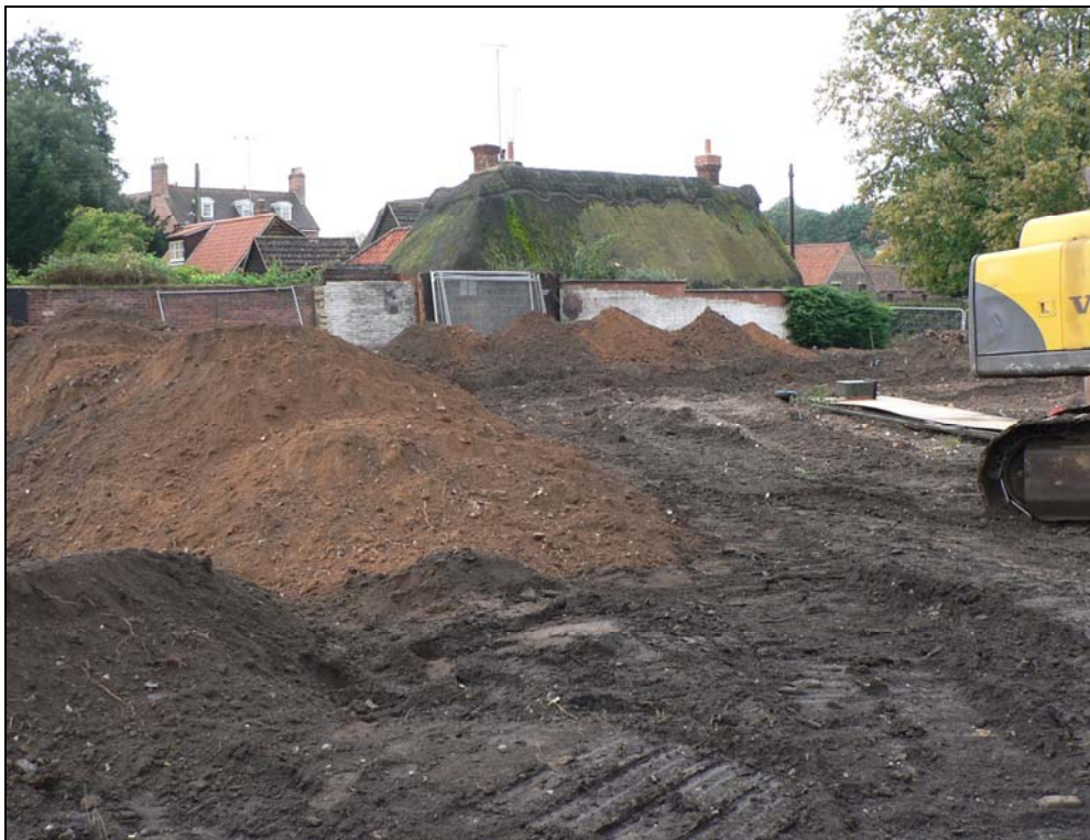
General view from northeast with listed building in background
