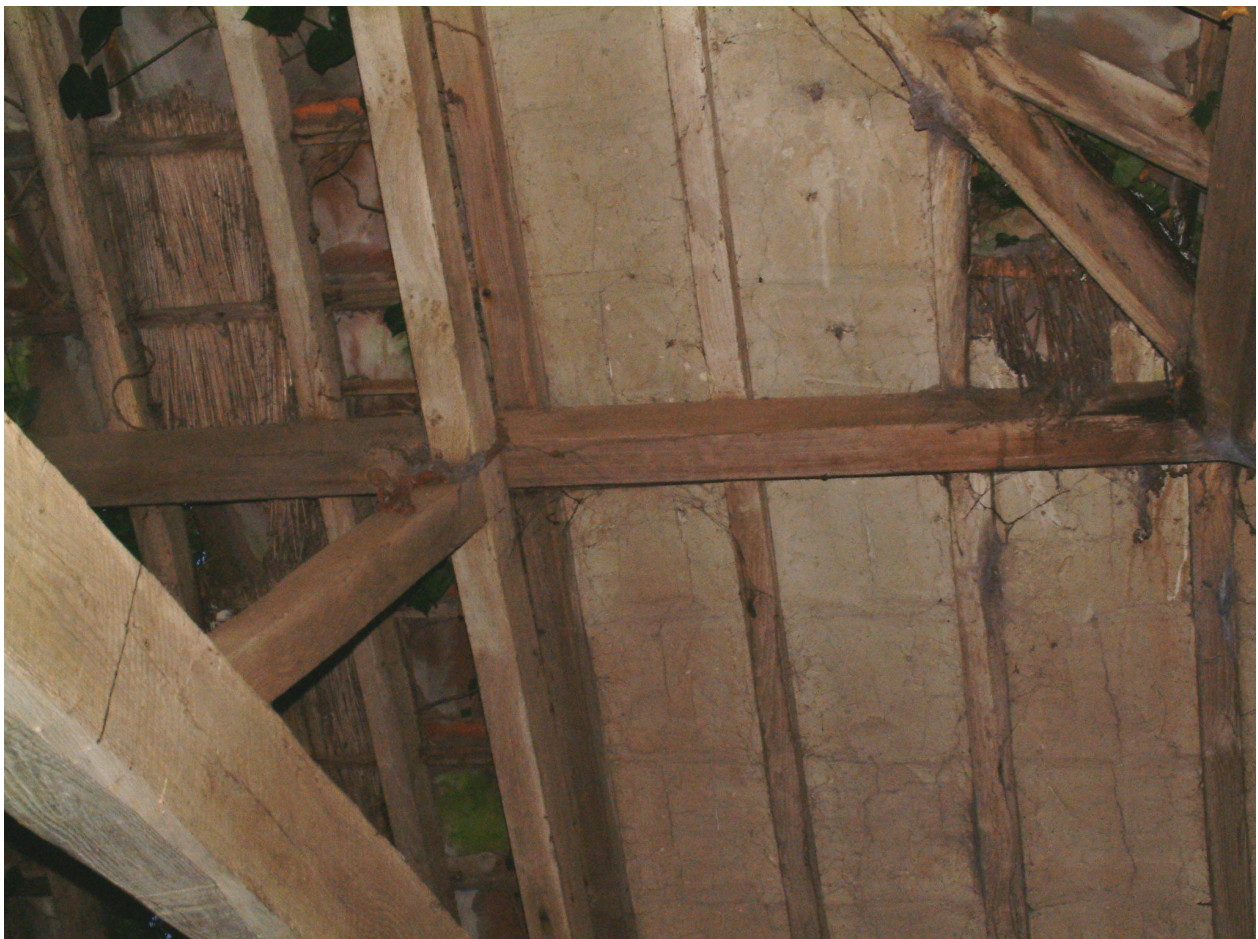
Photo 6.11 The plaster and reed undercoating of the pantiles
