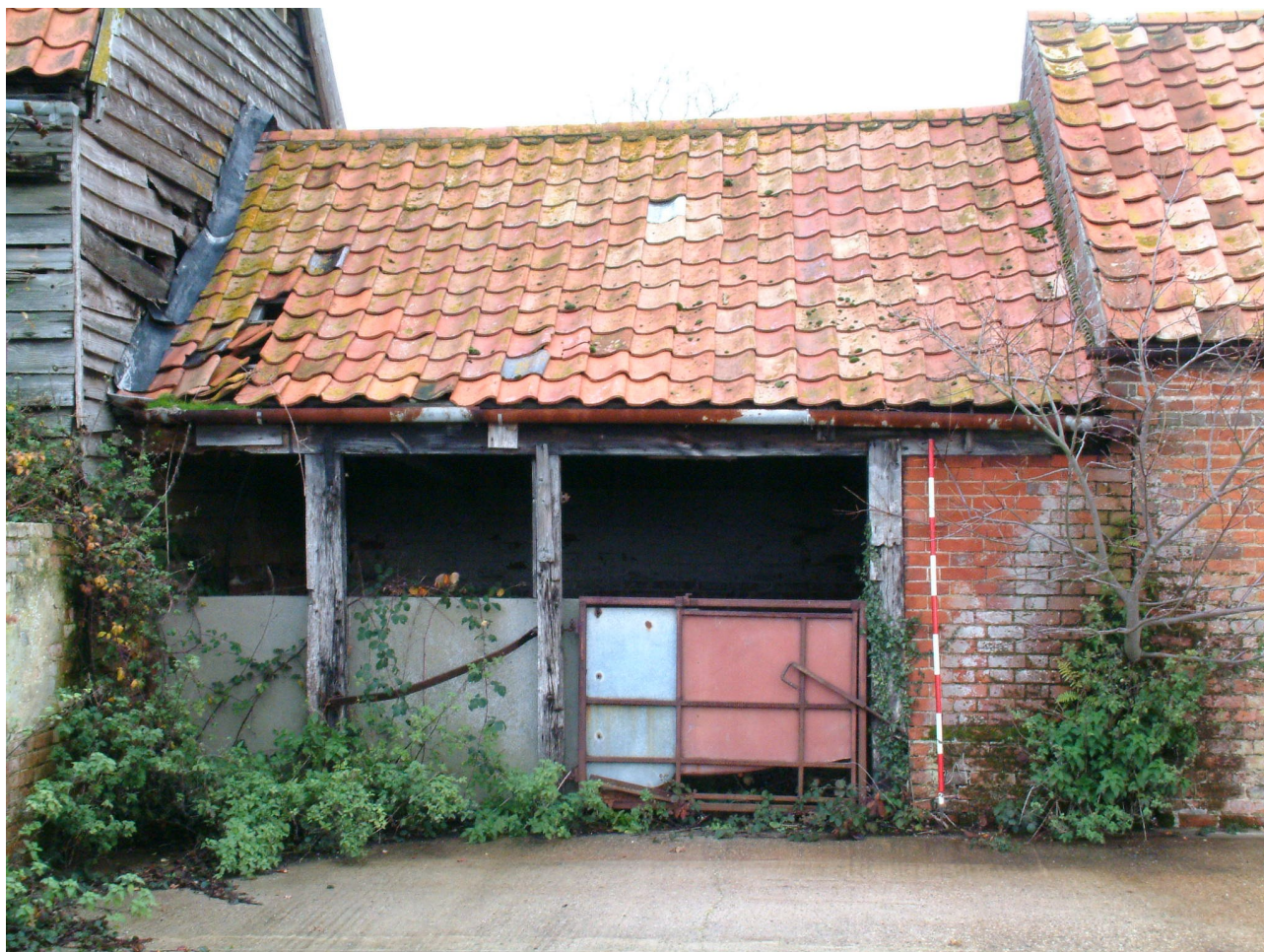
Photo 3.1 Later building inserted between the barn and Building 4
