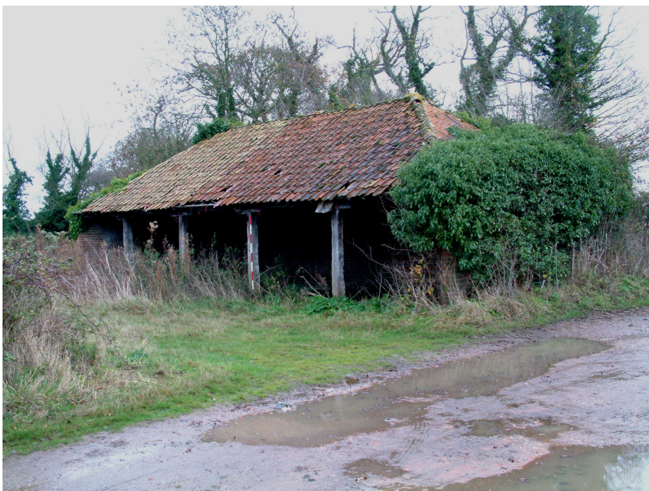
Photo 6.1 Shelter Shed from the south west
