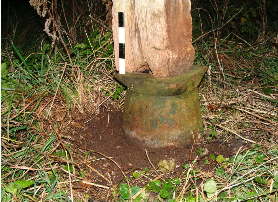
Photo 6.7 Iron pedestal supporting one of the western oak posts. 20cm scale.
