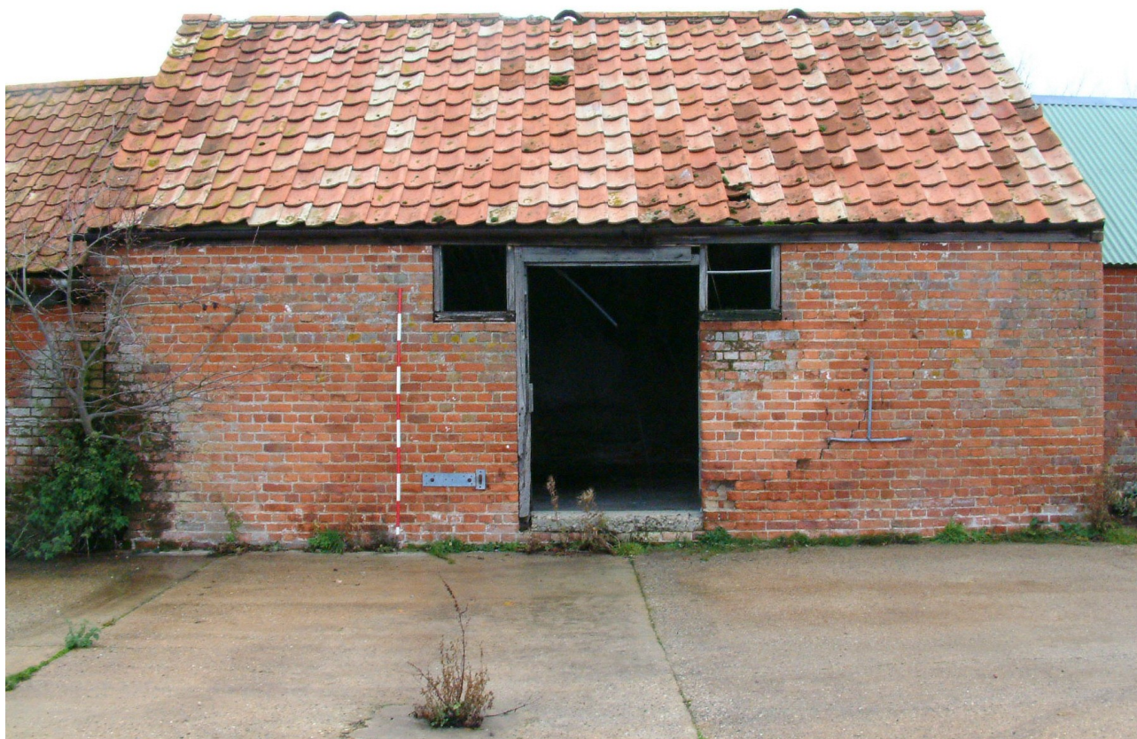
Photo 4.1 The south front of Building 4
