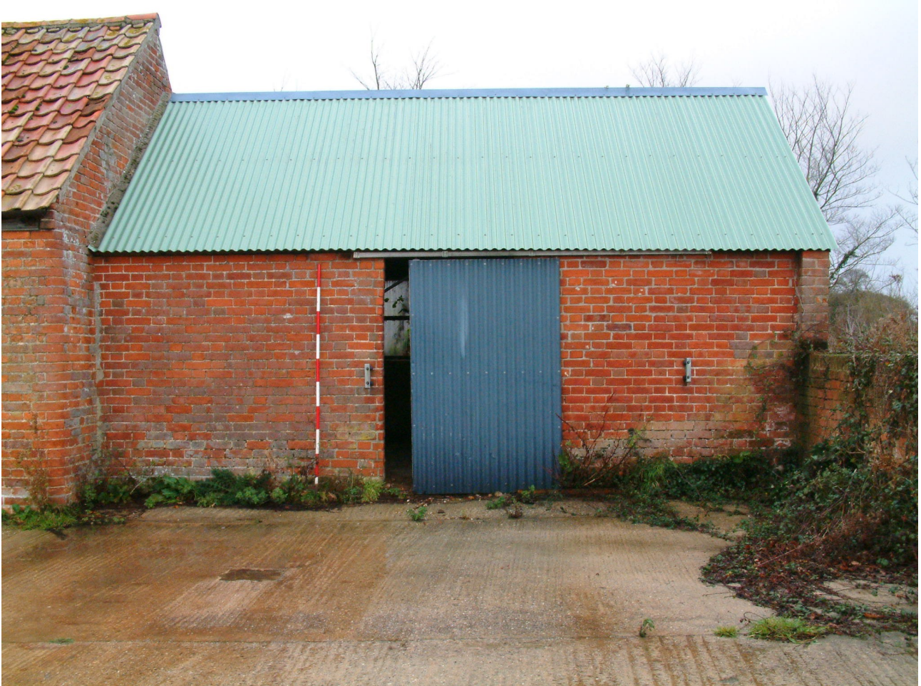
Photo 5.1 The southern annex, Building 5, from the south
