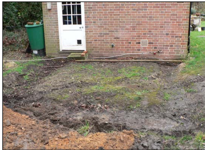
Extension area from west with northern and southern foundations in place
