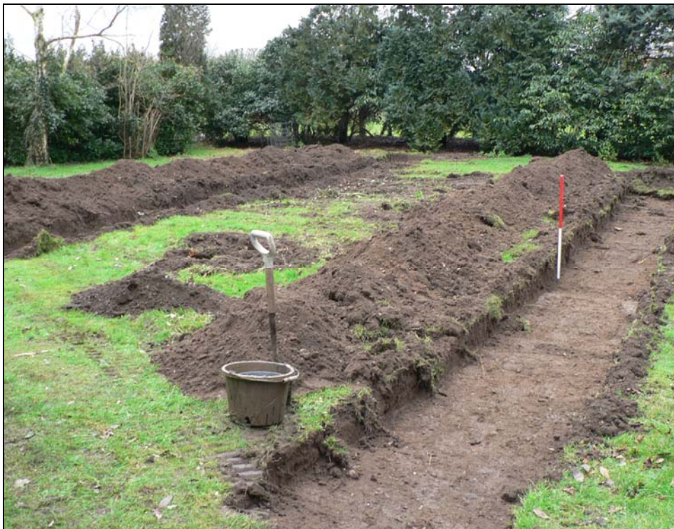
Access/parking area from northeast with trial trenches to formation level
