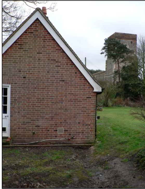
General view of extension area from west
