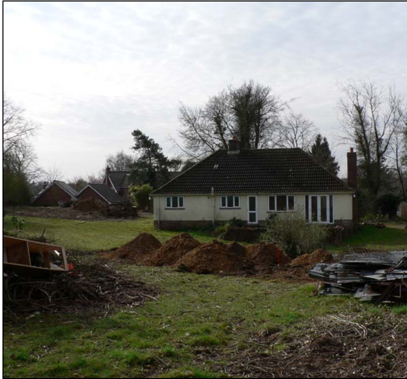
General view from north
