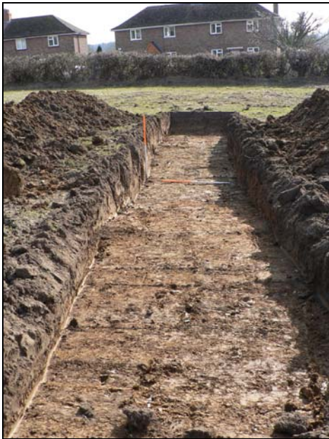
Trench 1 from north
