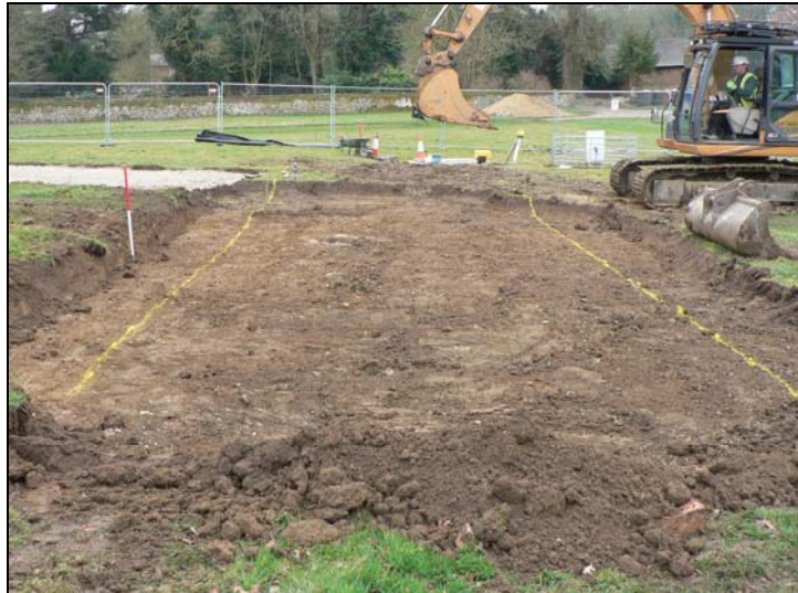
New tank area stripped of topsoil from north
