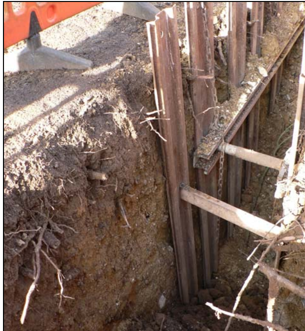
Pipe trench remedial work near the Porters Lodge
