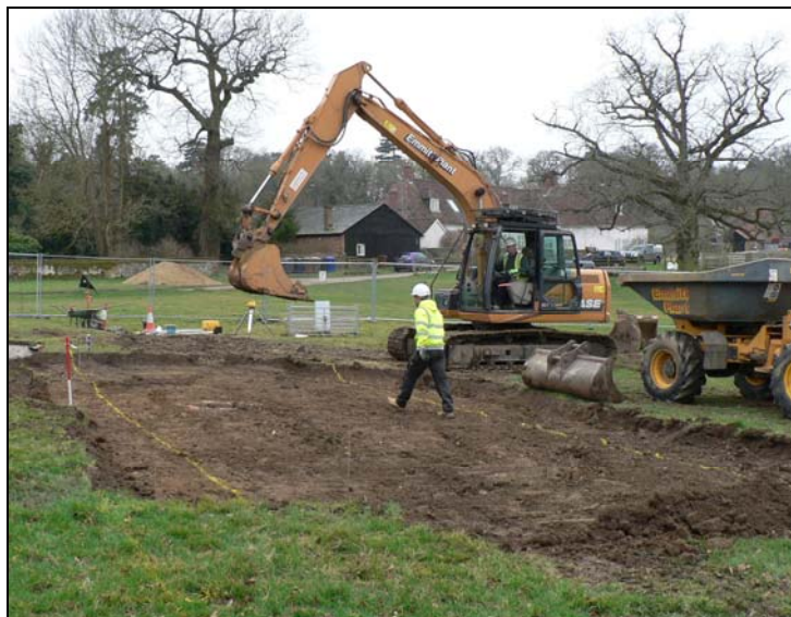
General view of new tank area from north
