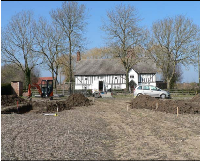
General view from south with Lodge Farmhouse in the background
