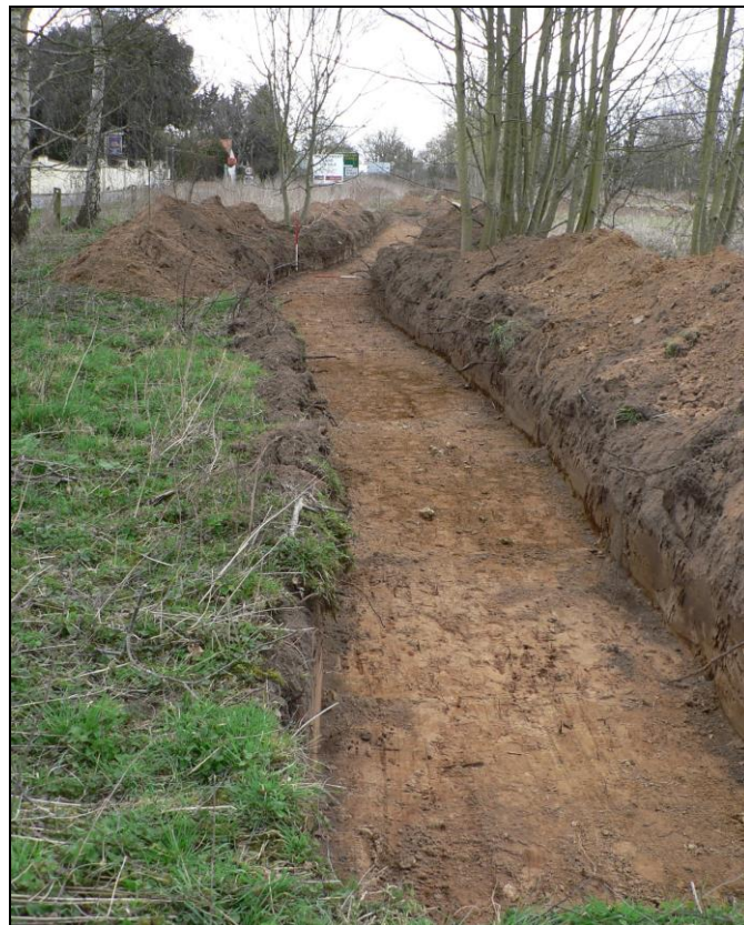
General view of typical trench (trench 3 on western side from south)
