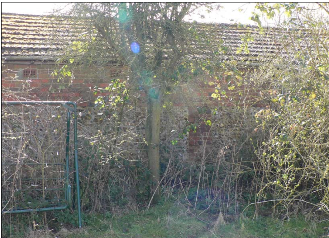
Northern wall of former 19 th C cart lodge from north
