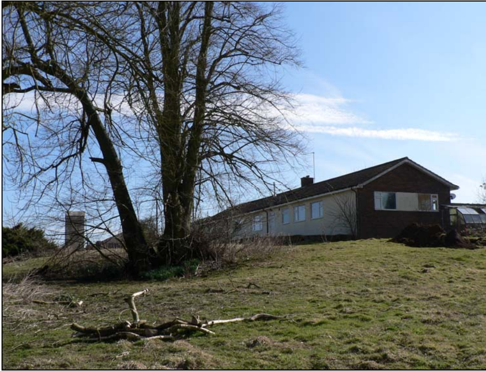
General view from north-west
