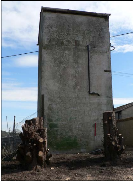
Water tower from west
