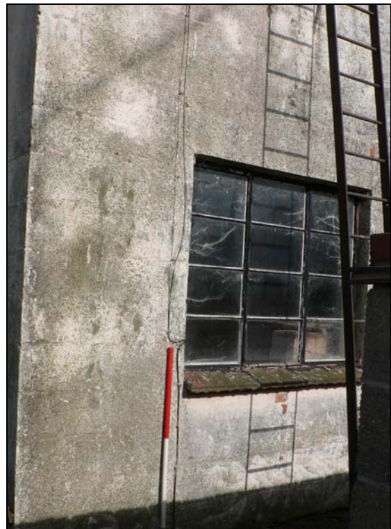
Water tower from south-west with detail of window
