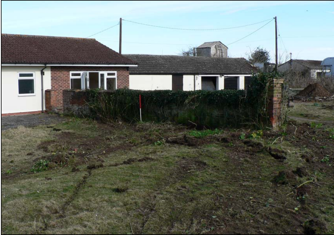
Brick 19 th century wall to front of bungalow from south-west
