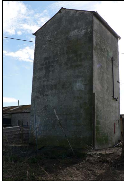
Water tower from north-west
