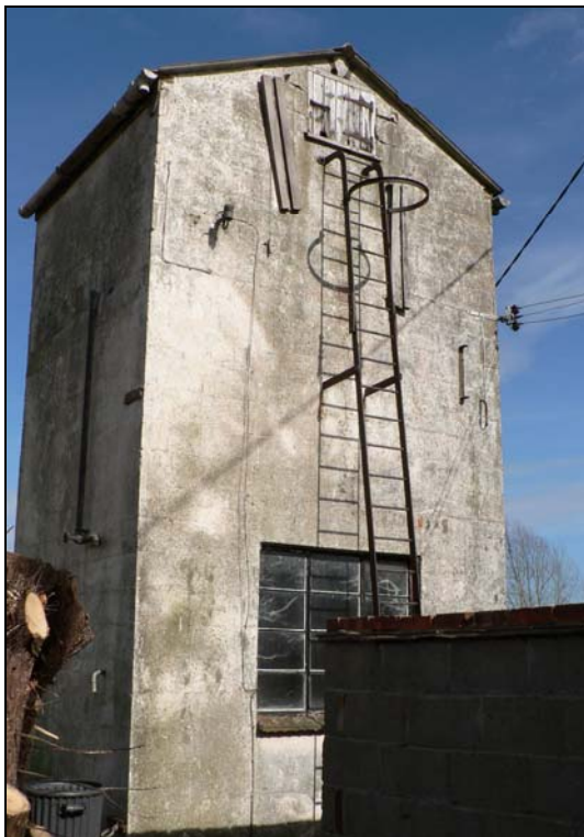
Water tower from south
