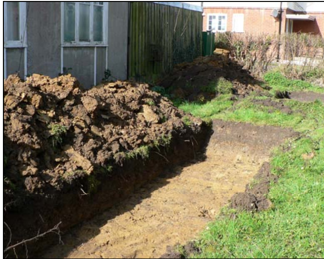
Eastern part of trench 1 from northeast
