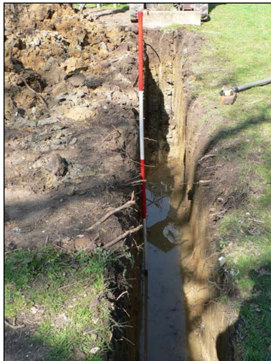
Northern trench from east
