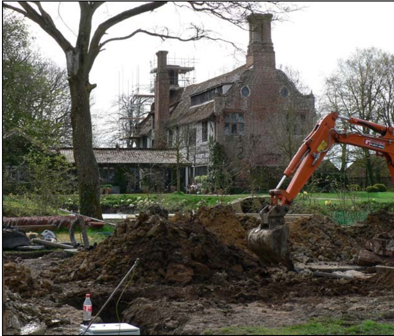
General view from west
