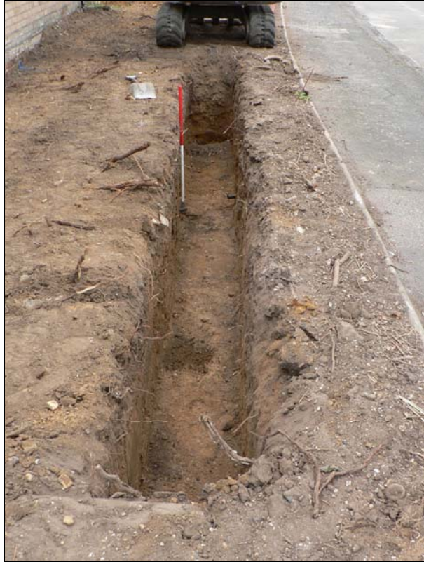
Side extension footings from south
