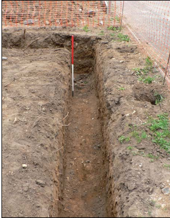
Garage eastern footing trench from south
