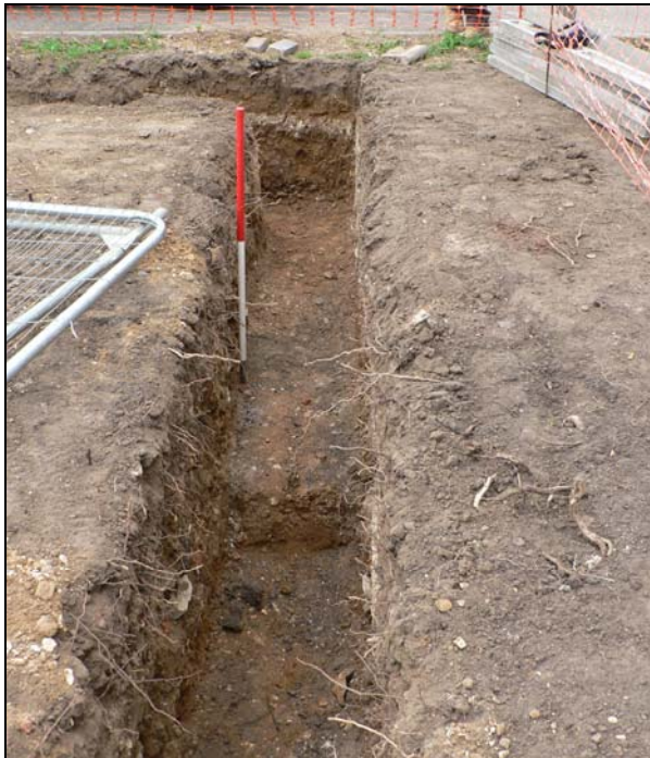
Garage northern footing trench from west
