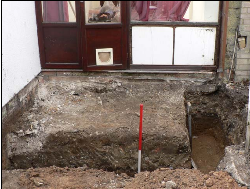
Small rear extension footings from south
