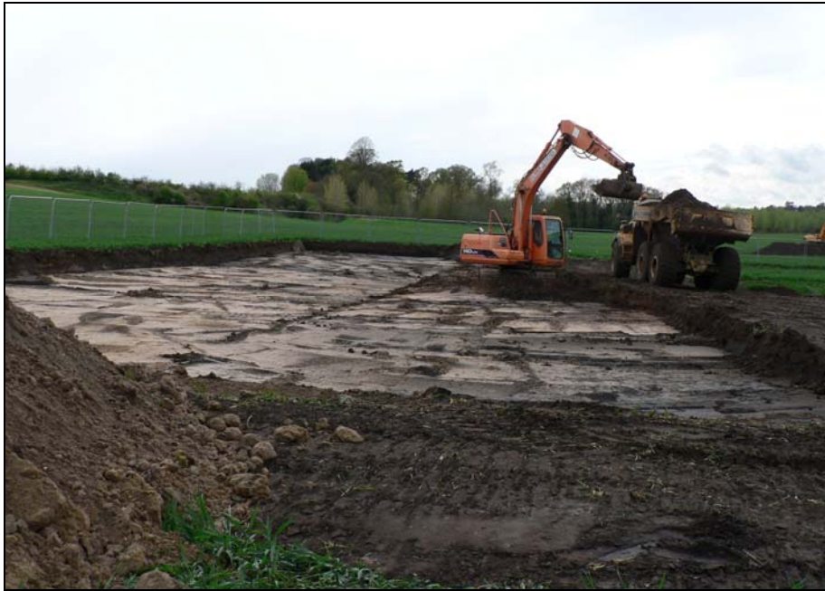
General view of monitoring stage from east
