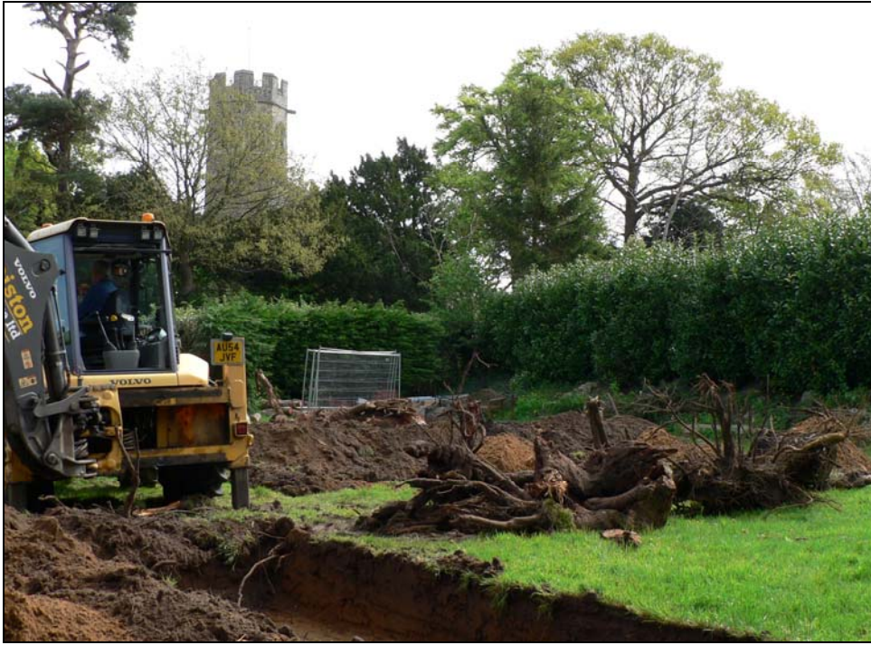
General view from west
