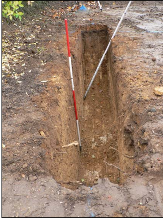
Monitored trench on western side of new house in the northern part of the site
