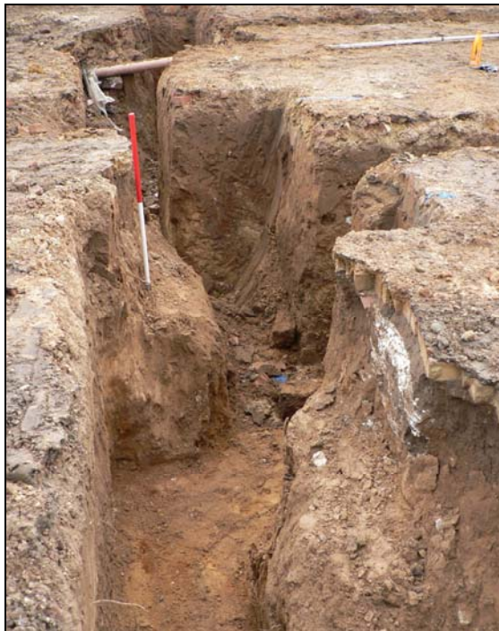
Monitored trench on northern side of new house
