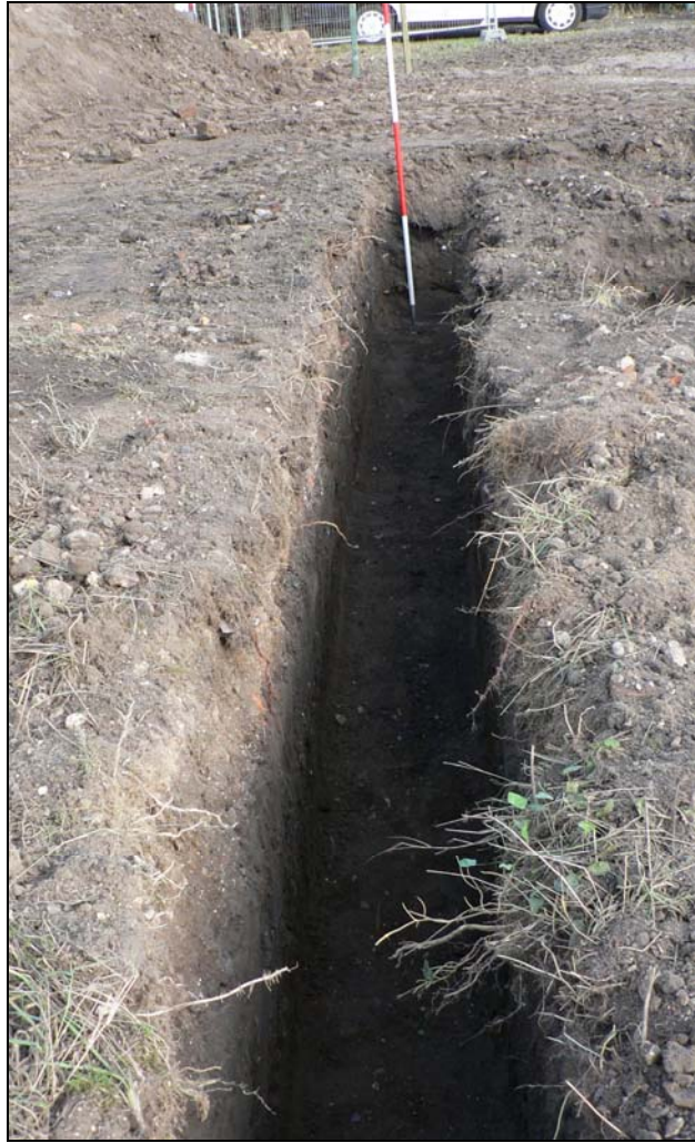
Northern footing from west
