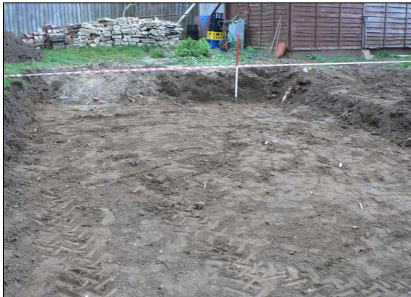
General view from south during initial soil stripping
