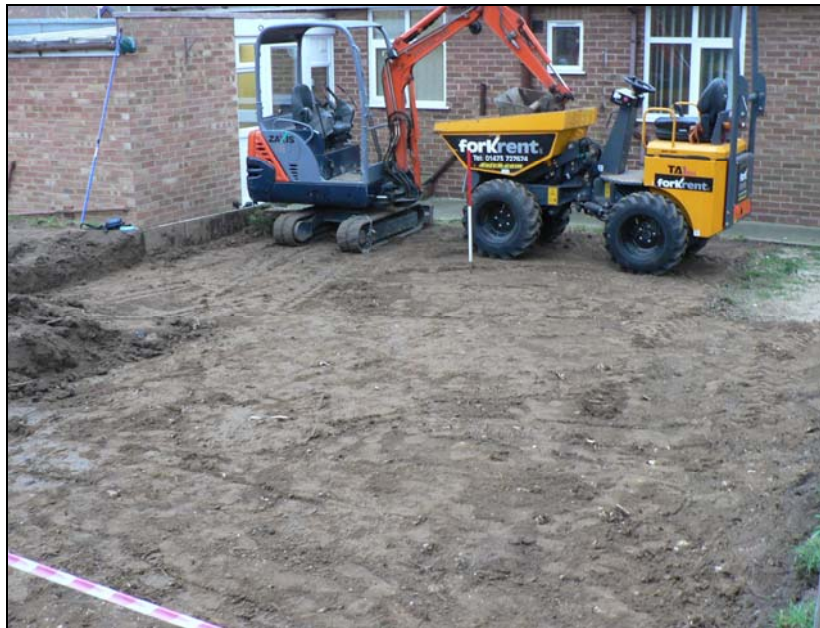
General view from north during initial soil stripping
