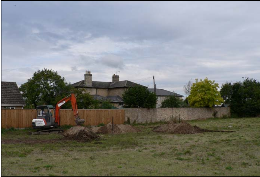
General view from southeast
