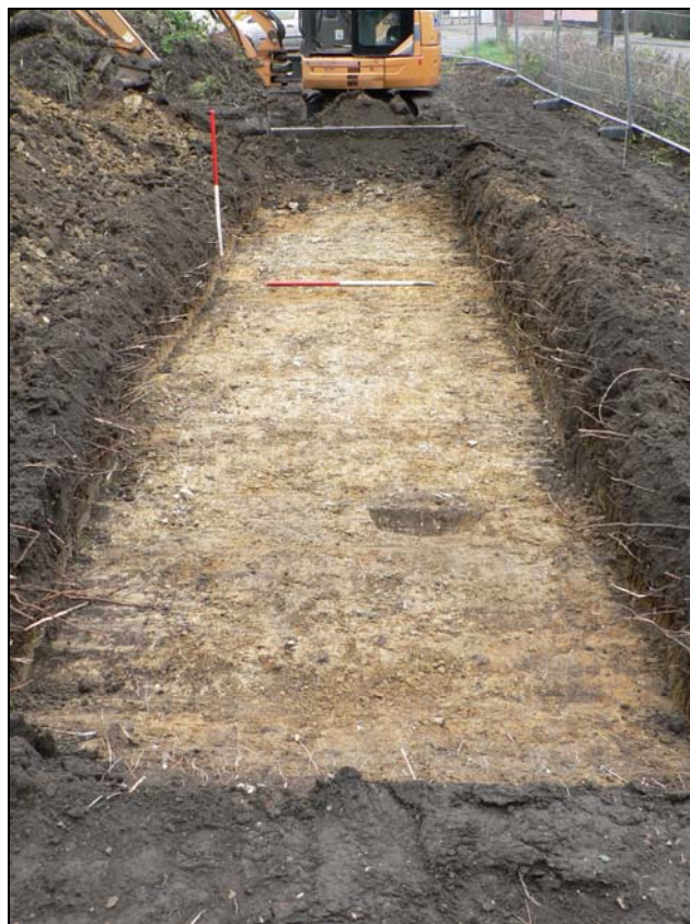
Trench from south
