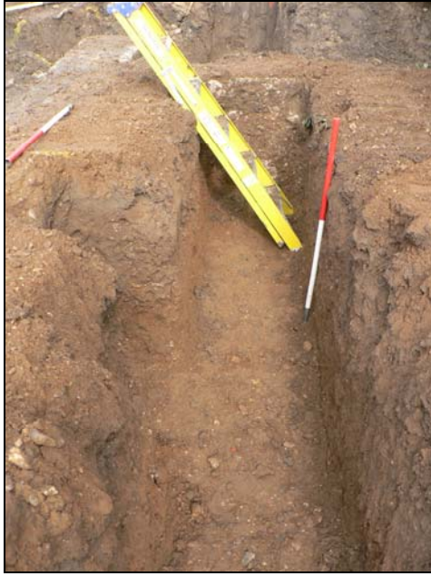
Eastern foundation trench from south
