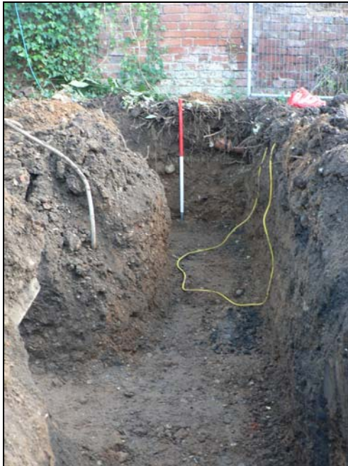
Southern foundation trench from east
