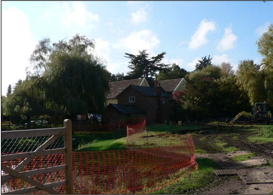
General view of annex area from northeast
