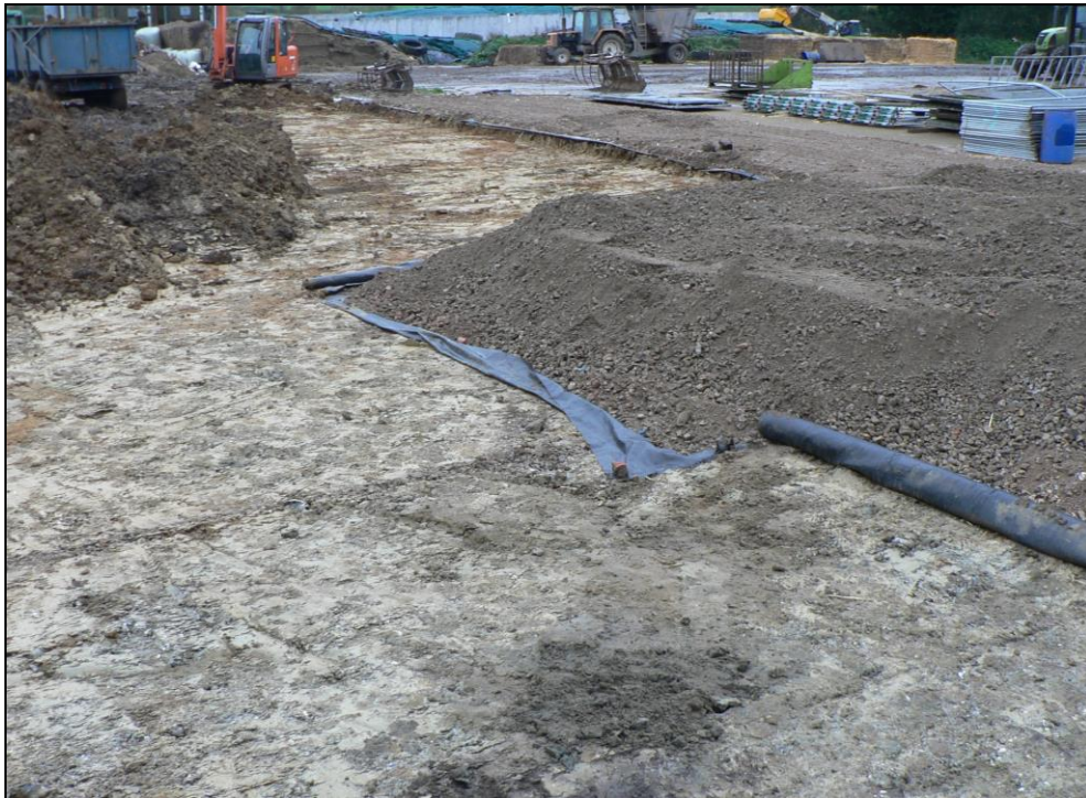
General view from north-east during soil stripping
