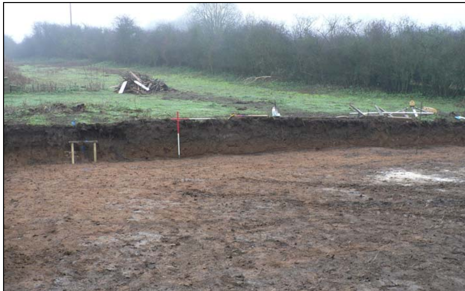
General view of initial ground lowering from southwest
