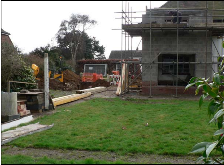
General view from north
