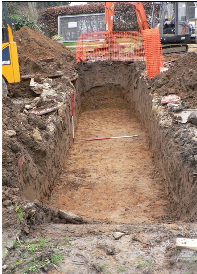
Trench 1 from north
