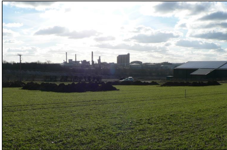
General view from northeast
