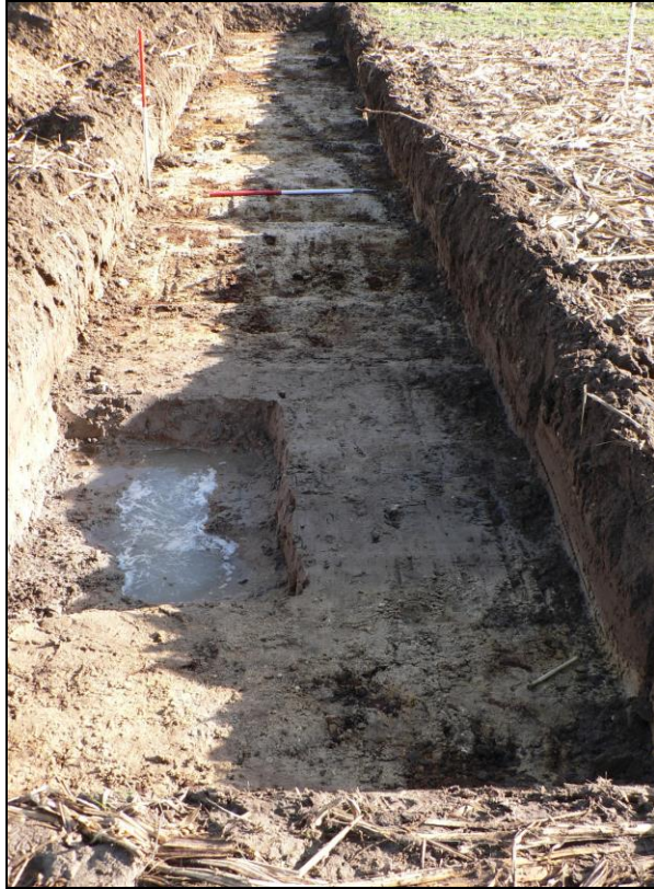
Trench 9 from west with tree root hole in foreground
