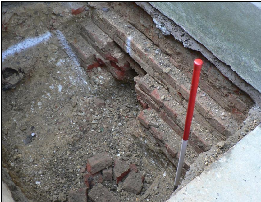
Pit in dry moat to front of west wing
