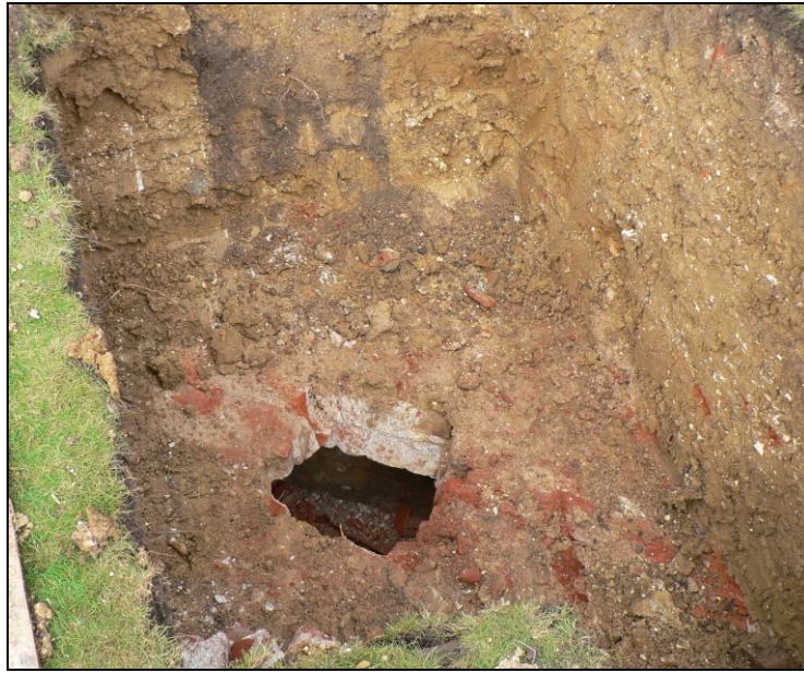
Brick culvert in Italianate garden to rear of west wing
