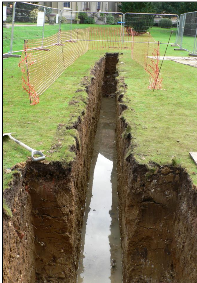
Trench to the rear of the west wing
