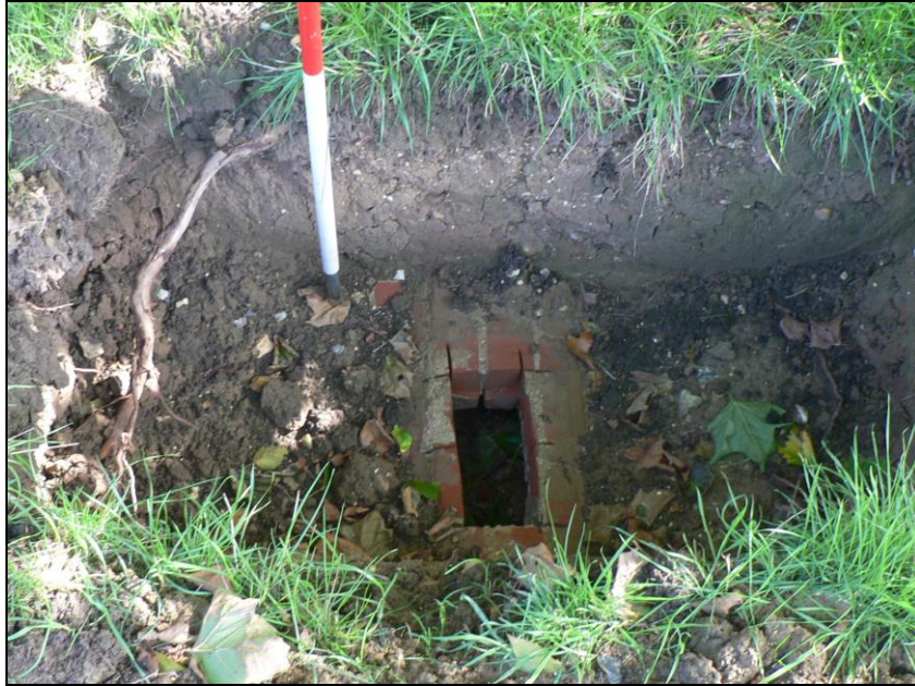
Brick culvert to west of Parsons Pond
