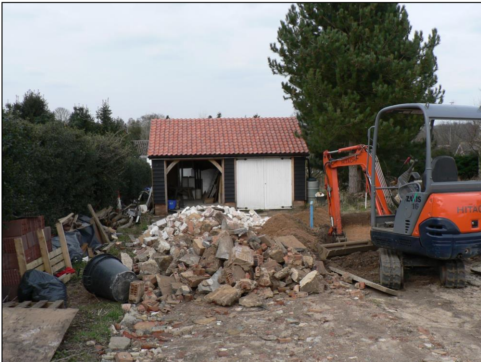
General view from south with new cart lodge
