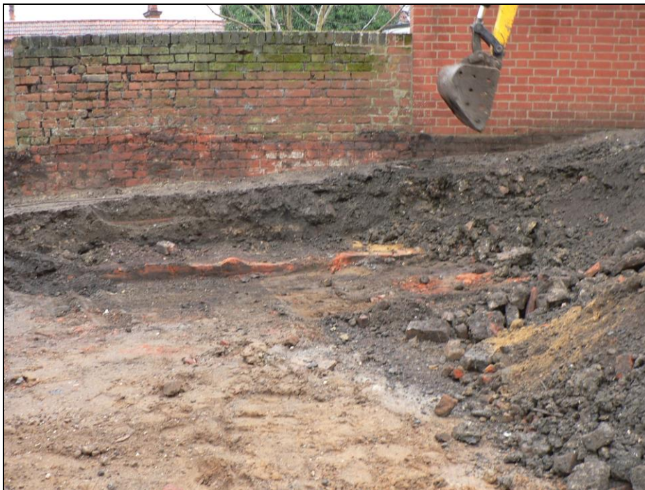
General view of soil stripping from west
