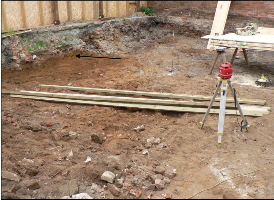
Base of raft foundation from southeast (subsoil deposit 0002 arrowed)
