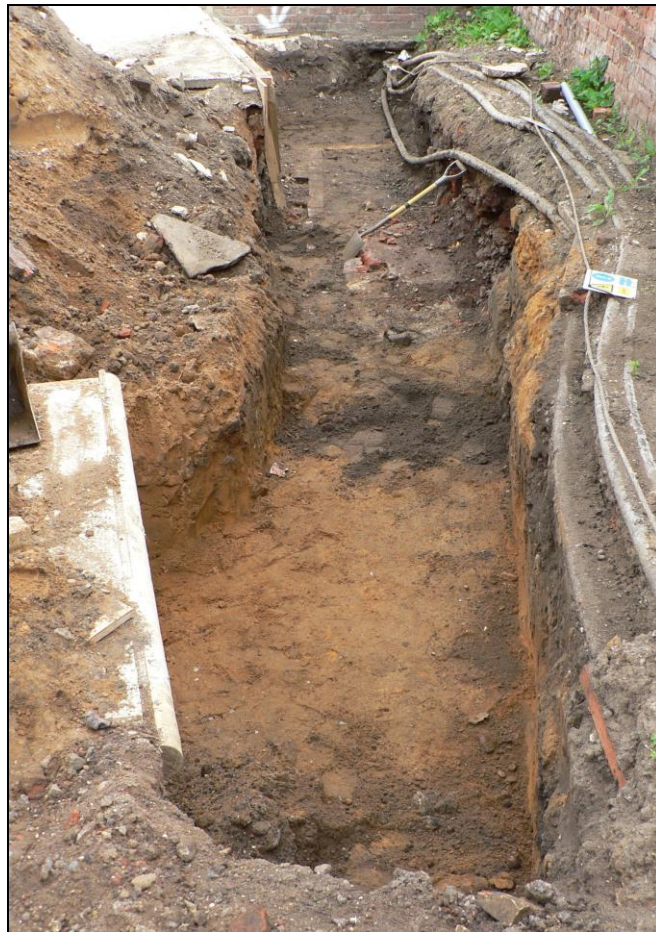
Cable trench from south
