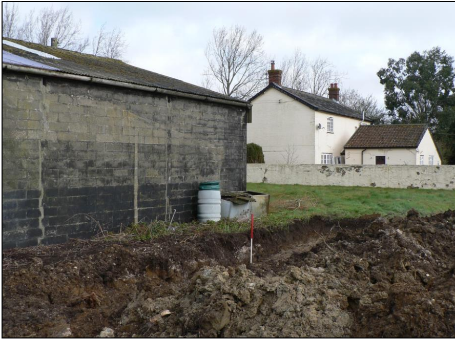
General view of from southwest towards Whitegates Farm House
