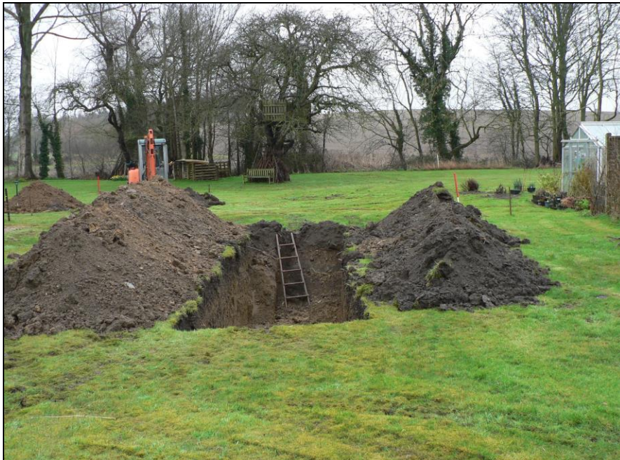
General view from south across trench1 (Chilton Stream beyond trees in distance)
