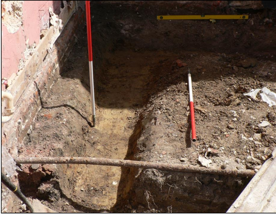
Raft toe at north-eastern end of extension area
