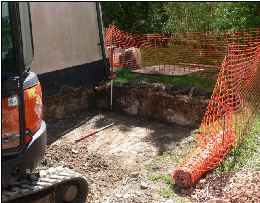
Sunken 19 th century brick floor in south-western part of new extension area
