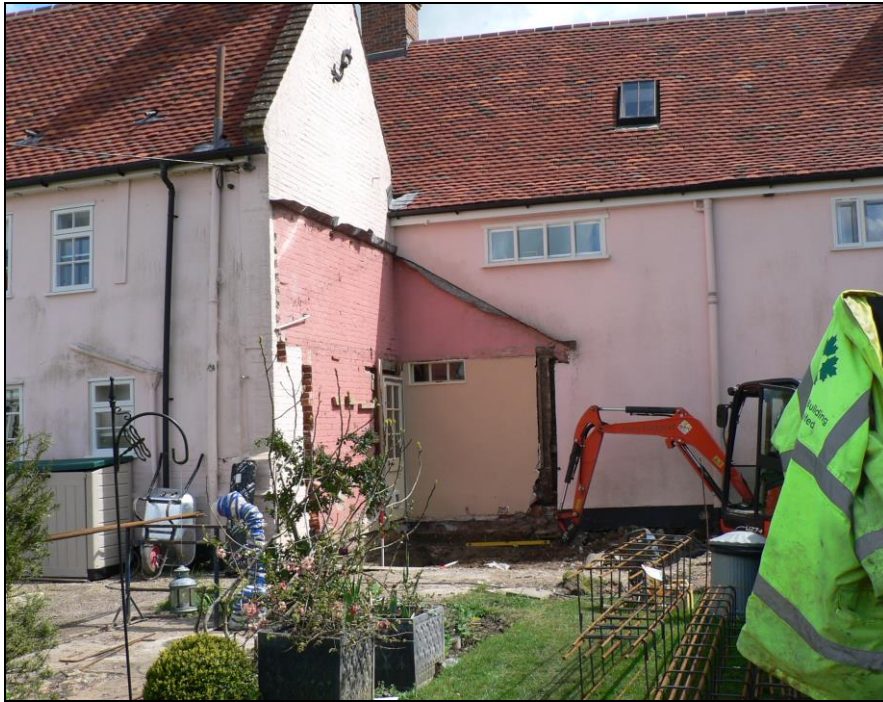
General view from north-west
