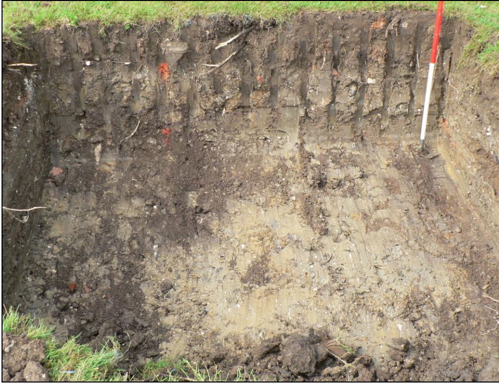
Deposit profile of treatment plant pit with recent brick fragments present to a depth of 600mm
