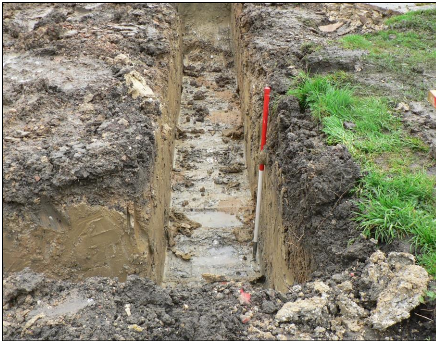
Trenches on southern side
