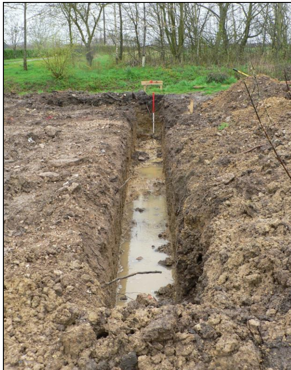
Eastern foundation trench from south
