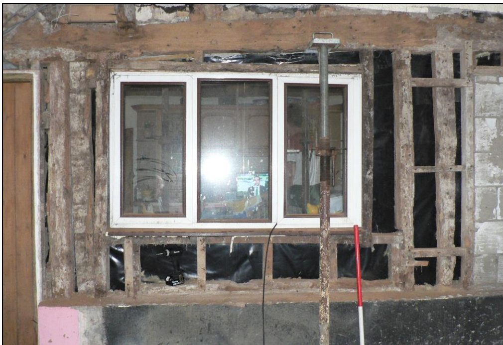
Detail of timber framing
