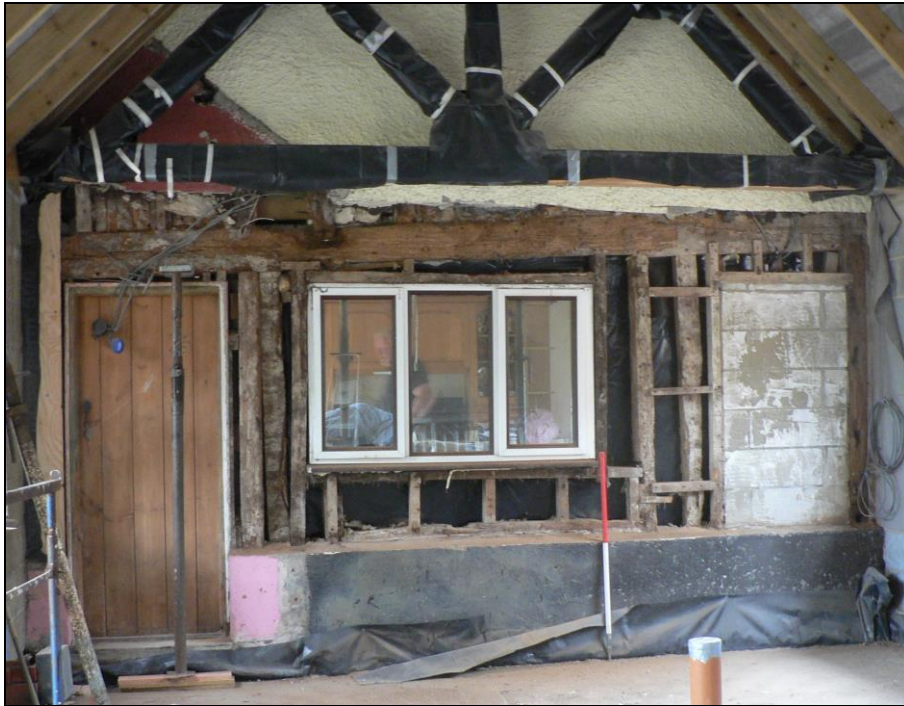
Eastern remaining timber framing exposed
