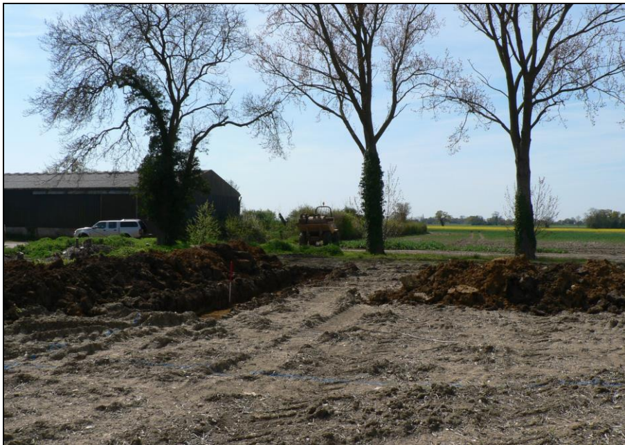
General view from north
