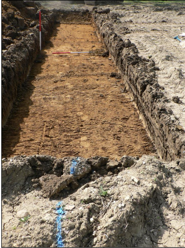
Trench 3 from north
