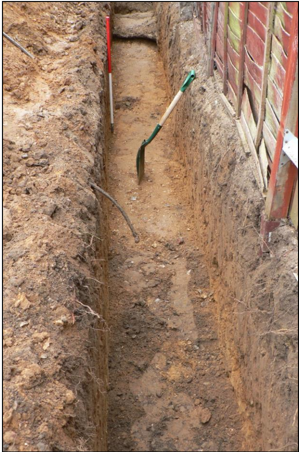
Western trench from north
