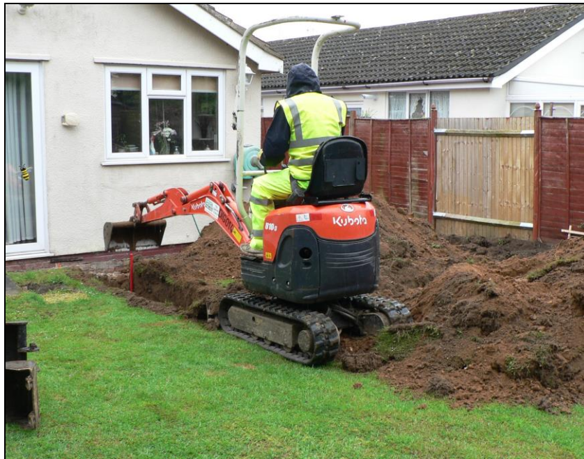
General view from north
