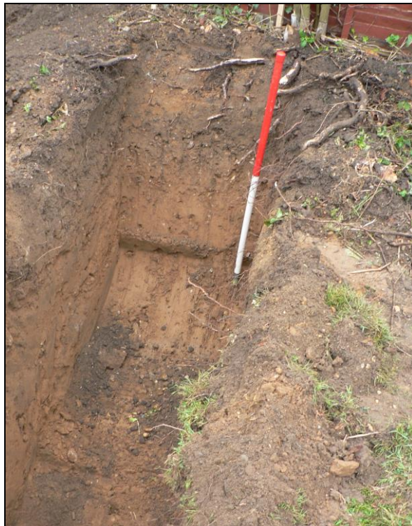
Foundation trench close to western boundary
