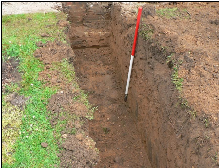
Foundation trench close to the rear of the house
