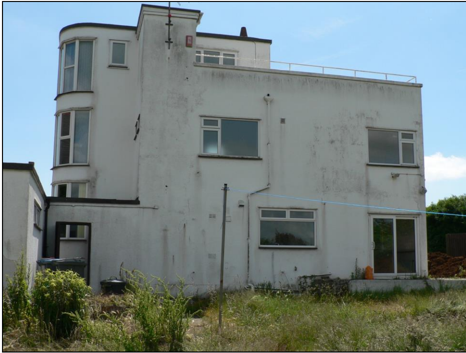
General view of house from north
