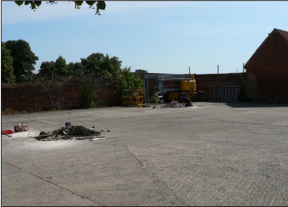
General view of yard area from northwest
