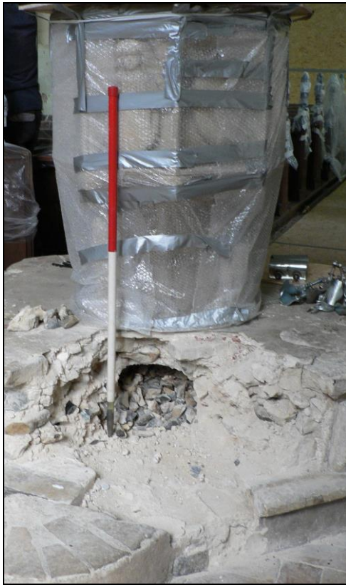
Investigation of font base with loose flints in the core
