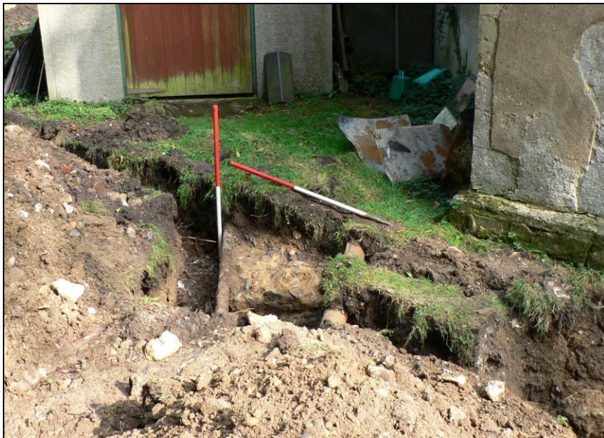
Early flint and mortar foundation 0003 to north-west of church
