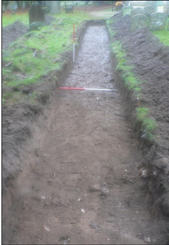
Trench arch drain from east
