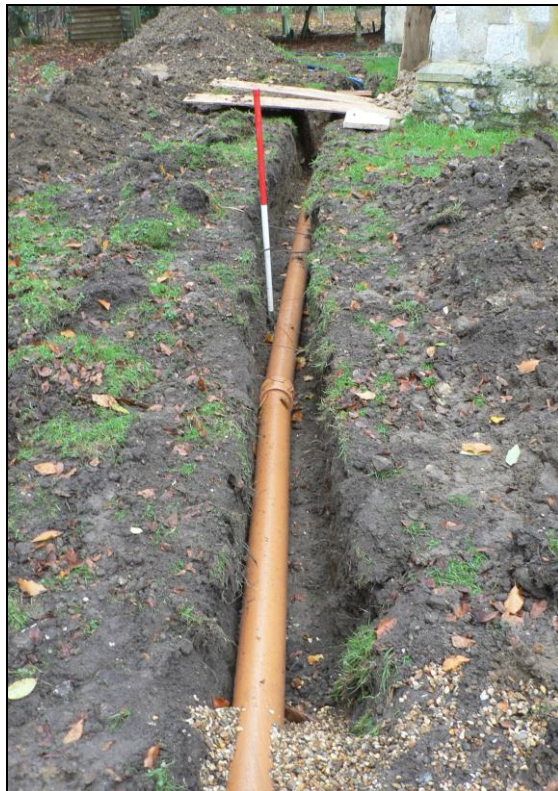
Pipe trench to south-west of church
