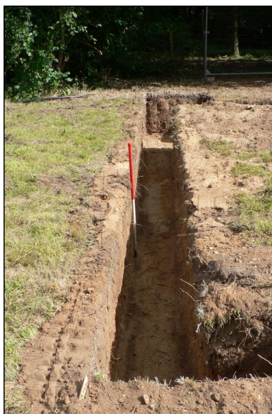
Northern garage foundation trench from west
