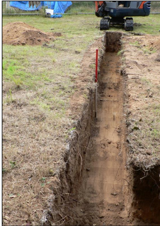
Southern garage foundation trench from east
