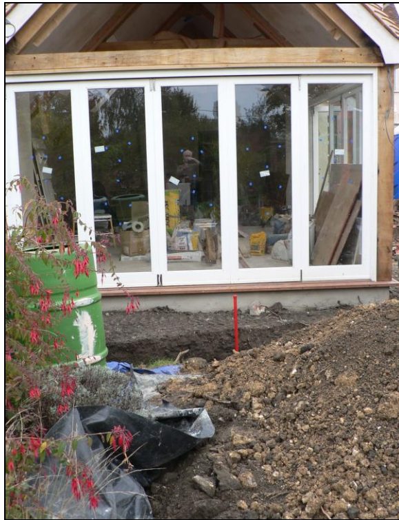
General view from west
