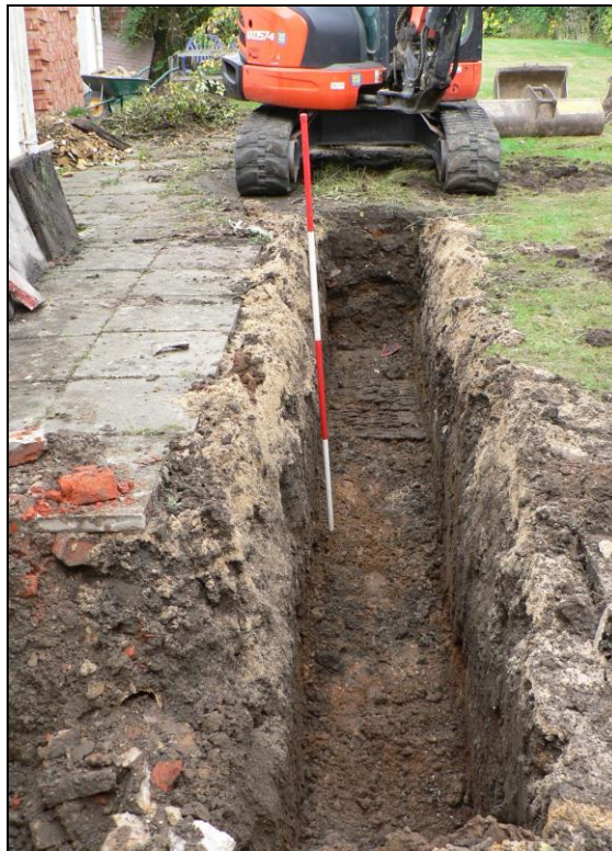
Southern trench from east
