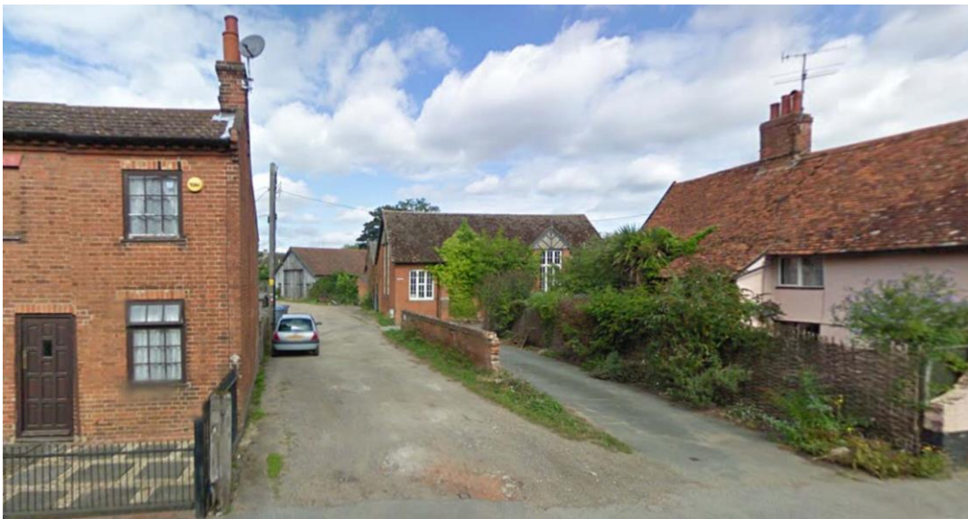
Fig. 1 Double vehicular access from The Street looking west
