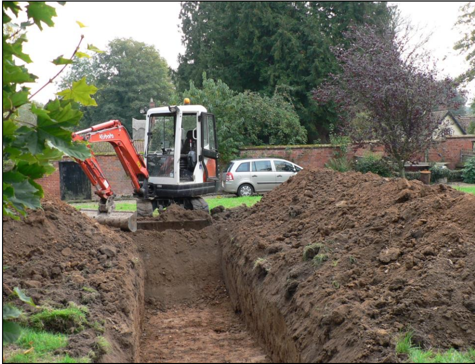
General view from north
