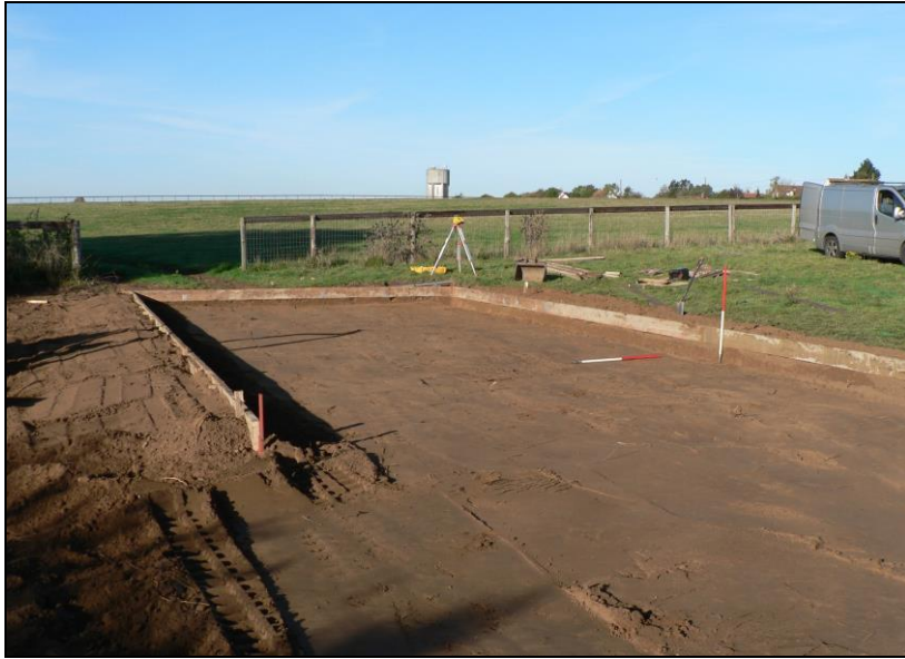
General view of stripped area from east
