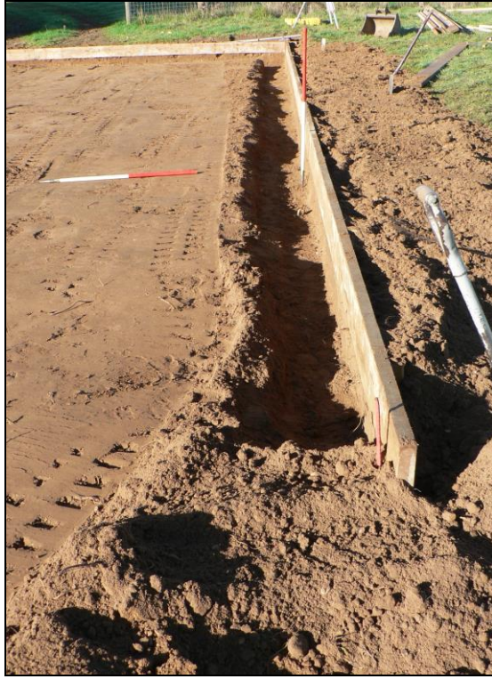
Stripped area and northern raft toe
