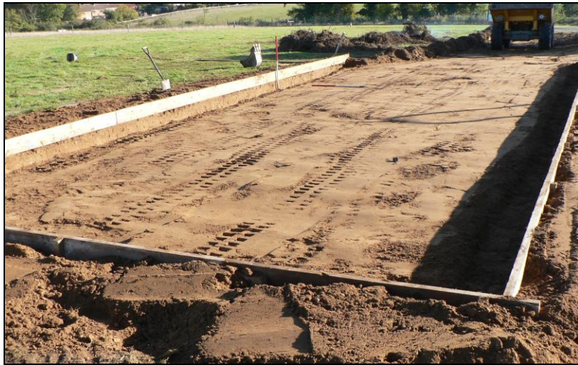
Stripped raft area from southwest
