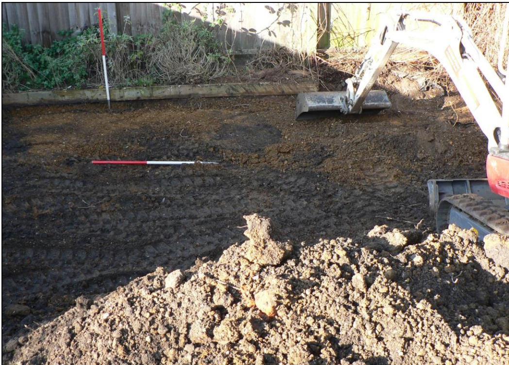
Stripped raft foundation area from east
