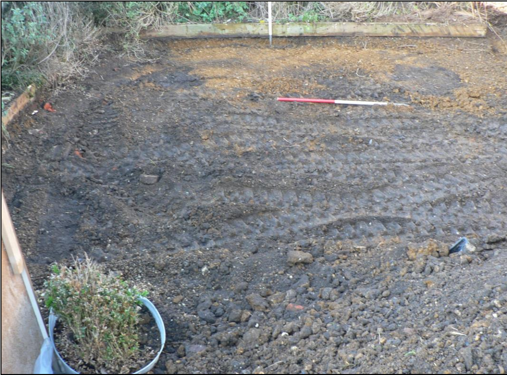
Stripped raft foundation area from south
