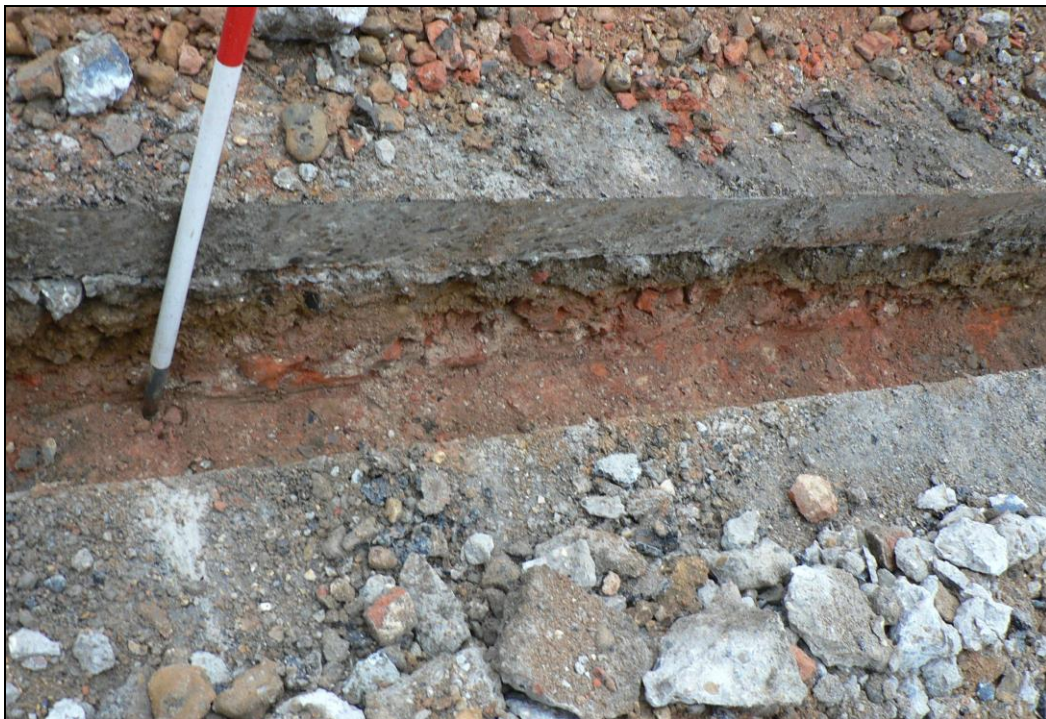
Brick wall foundation/floor 0010 just inside entrance to park at gate house
