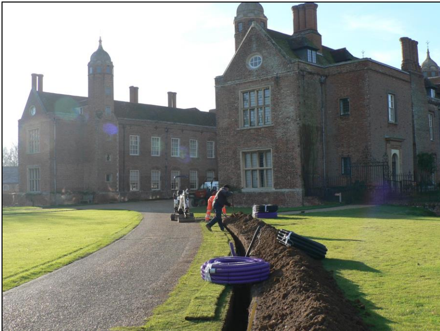
General view of cabling works from northwest
