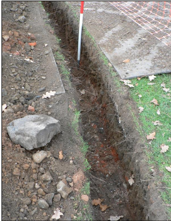
Possible brick wall foundation running along side of trench
