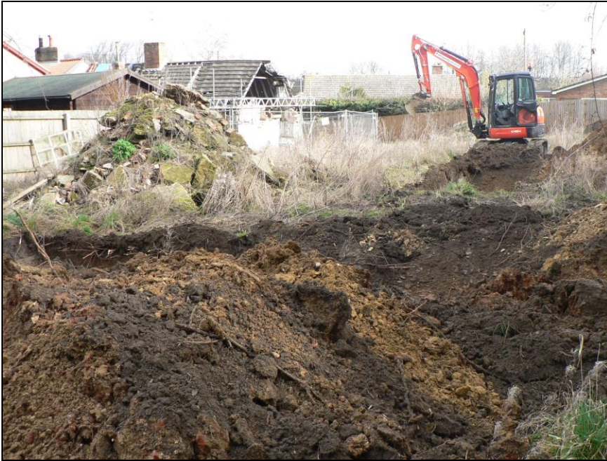
General view from west
